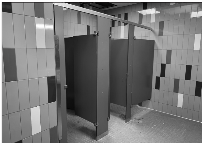
The restroom remodeling is almost complete!
